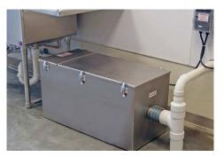
provides requirements for sizing and installing a grease trap.
